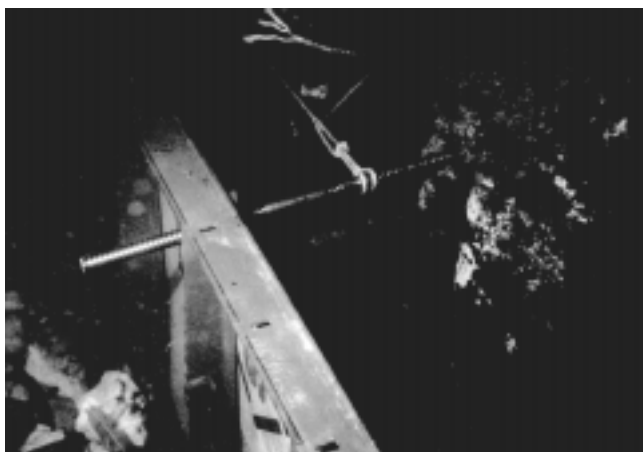
Fig. 5.1—"Symonds" forms in place underwater for pumped repair. (Courtesy of M. Garlich.)
