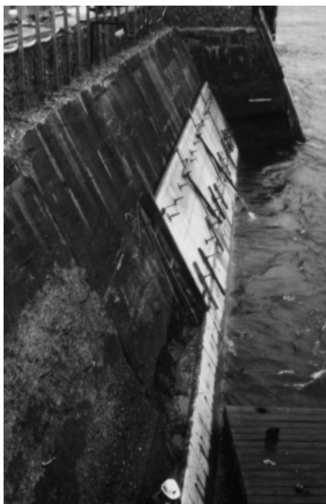
Fig. 5.2—Lower of three tiers of panels used to overlay the Troy Lock river wall were placed and infilled under partially submerged conditions. (Courtesy of J. McDonald.)
